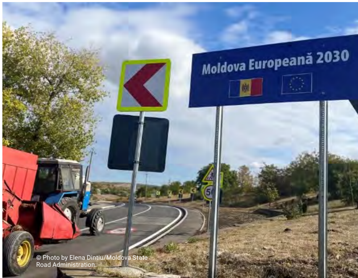
Figure VII. The renovated road in Chistelnita with modernized road safety infrastructure.
